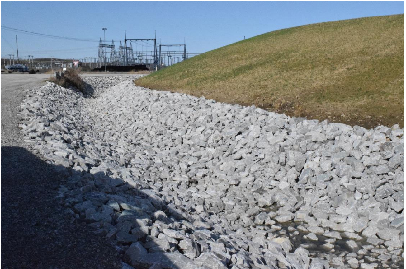
Southwest corner – lined ditch
