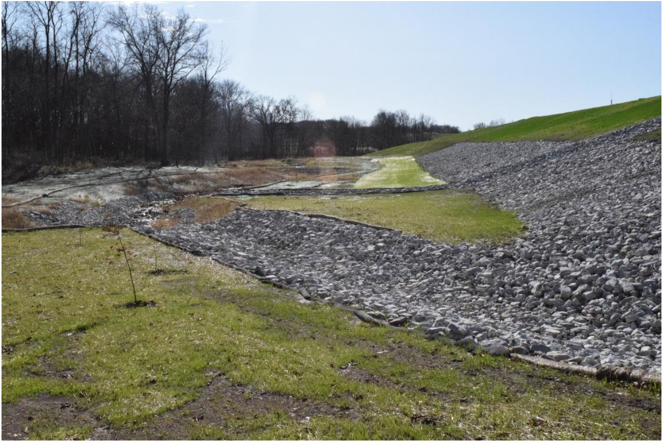
East toe area
